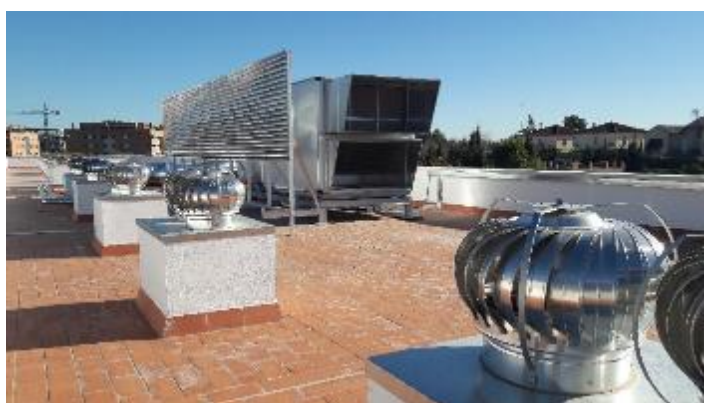
Figure 73 – Roof stacks connected to each classroom to increase the cross-ventilation rate
