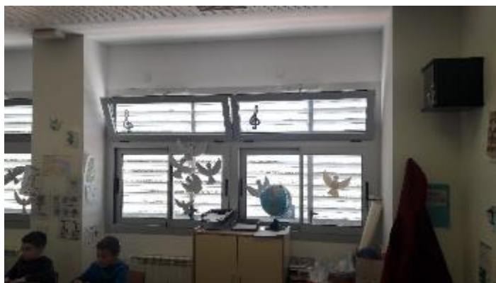
Figure 72 – Smart windows openings through CO 2 concentration sensors
